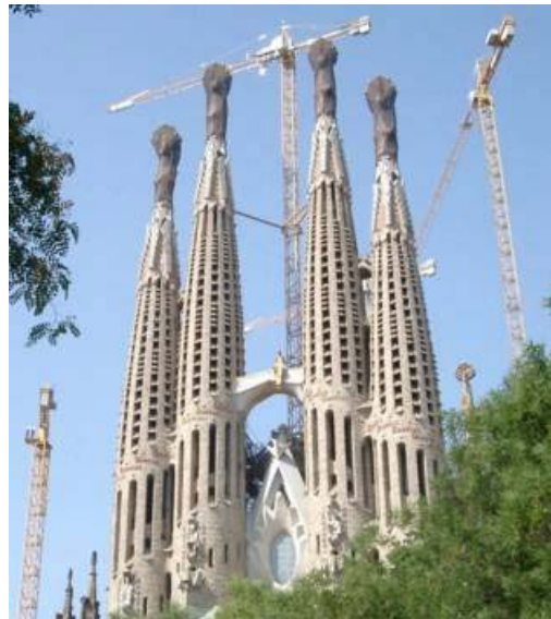
Figure 1. Cranes at la Sagrada Familia in Barcelona
