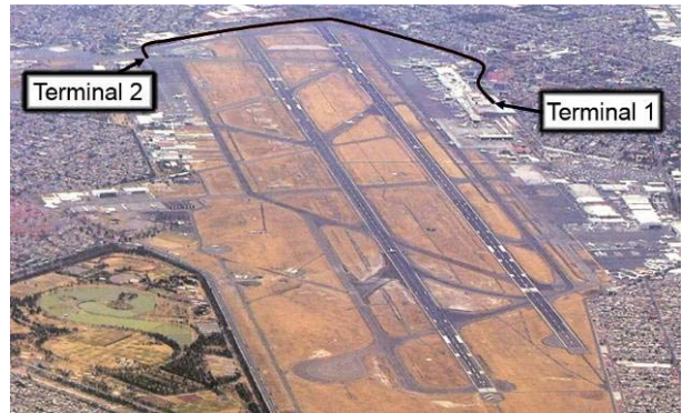
Figure 17. International Airport, Mexico City [10]
