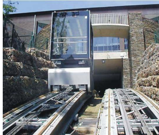
Figure 20. Inclined lift, Spa, Belgium [10]
