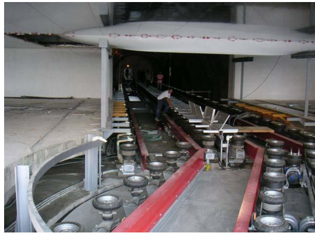
Figure 24. Rotating platform in the end station during the construction work [6]
