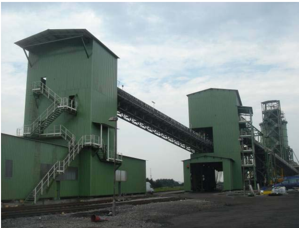
Figure 1. Two Rail load out building
