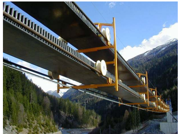
Figure 10. Detail view with track rope support frames and wheels rollers
