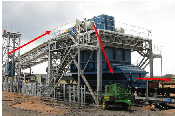
Figure 2. Transfer chute – material flow in same direction
