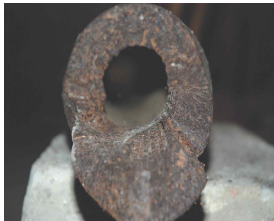
Figure 4. Photo of section in which there was a fracture of pipe.
