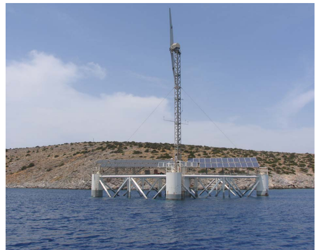
Figure 10. Floating wind turbine configuration. [Author's research]
