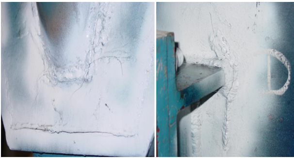
Figure 6: Example of cracks of the steel structure of the roller mill.
