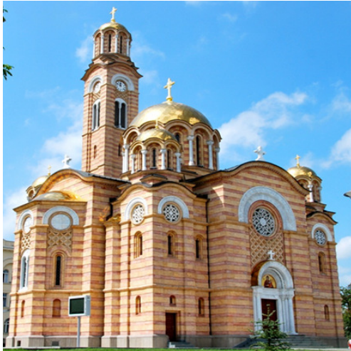
Figure 1: Cathedral of Christ the Saviour in Banja Luka, built in 1925, rebuild in 2004.
