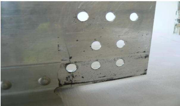
Figure 18. Wall crack path
