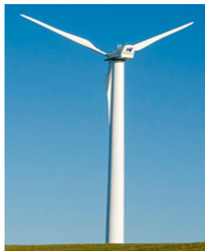
Figure 2. Wind turbine (WindPACT 1.5-MW) [4].
