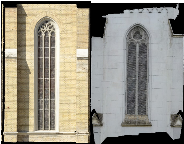
Figure 4. Orthophotos of the windows, obtained by using photogrammetry
