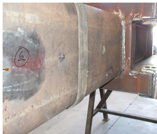
Figure 26: Install the strain gauges both inside and outside the sheet to compare the readings.
