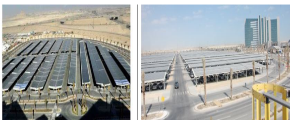
Figure 8. Photo of a 10 MWp installed capacity grid-connected PV power plant in Saudi Aramco, Dhahran, Saudi Arabia [17]
