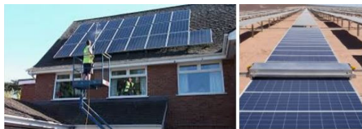
Figure 18. Manual and robotic cleaning (large PV plant) demonstration photos
