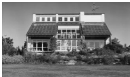
Figure 14. A grid-connected BIPV under 100,000-Roof-Solar-Programme in Germany [81]
