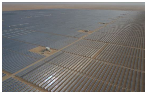
Figure 11. Sakaka solar power plant [17].
