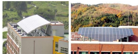
Figure 9. BIPVs installed in Dongo Elementary School (Left) and Osan Building (Right), [41]
