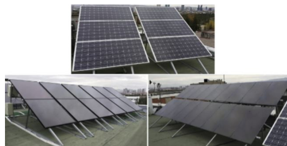
Figure 15. Grid-connected BIPV systems (mono-silicon, monocrystalline, and CdTe) installed and tested in Anatolian, climatic conditions [85]
