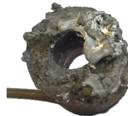
Figure 11. Failure mode by excessive corrosion of the heating set incapacitating the coil heater.
